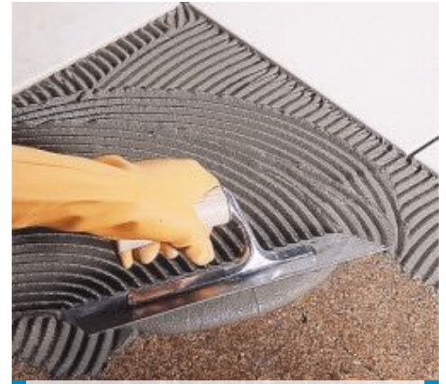
Installation of single-fired tiles on cork
