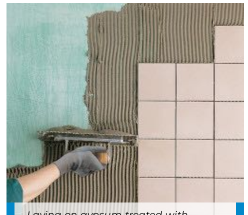
Laying on gypsum treated with Primer G
