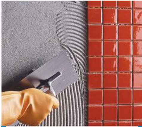
Installation of mosaic ceramic on wall
