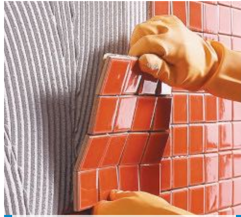
Installation of mosaic ceramic on wall
