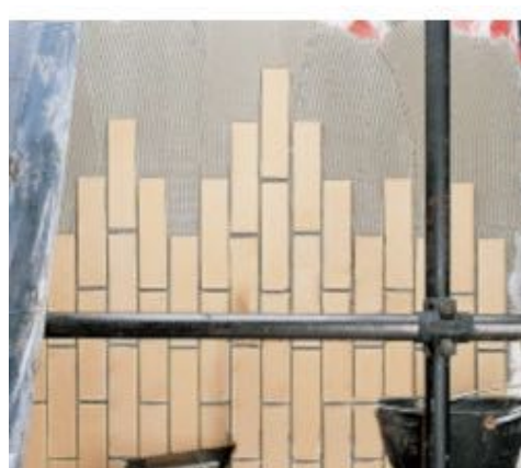
Exterior wall fixing
