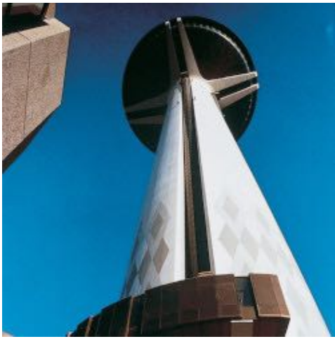
Porcelain tiles laid with Kerabond + Isolastic - Civic Center - North York Ontario (Canada)
